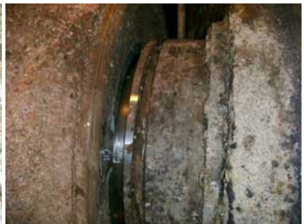
WEAR DOWN GAUGE 量測
