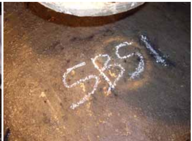
No.1 WBT(S) stripping bellmouth underside
