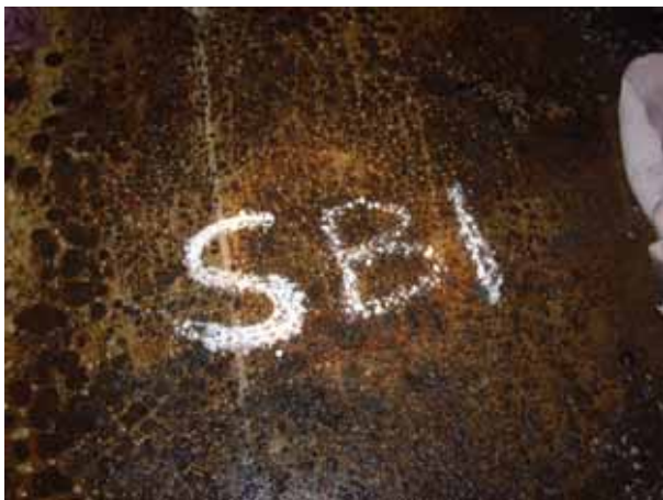
No.1 WBT(S) Bellmouth underside
