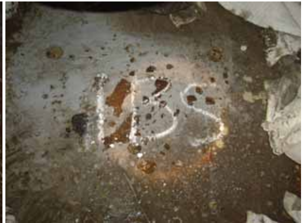
No.1 WBT(P) stripping bellmouth underside
