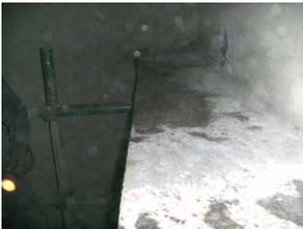
NO.1 P WBT CHIPPING AREA
