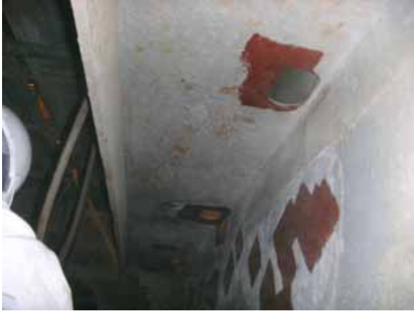
NO.1 P WBT CHIPPING AREA
