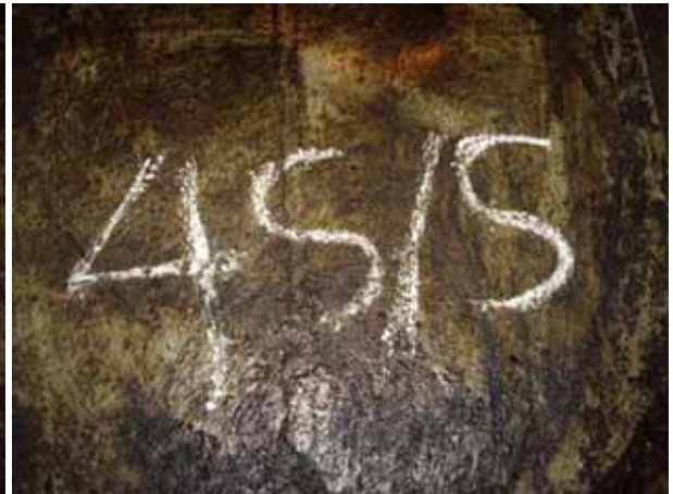
4S stripping bellmouth underside
