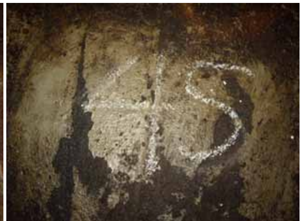
4C stripping bellmouth underside
