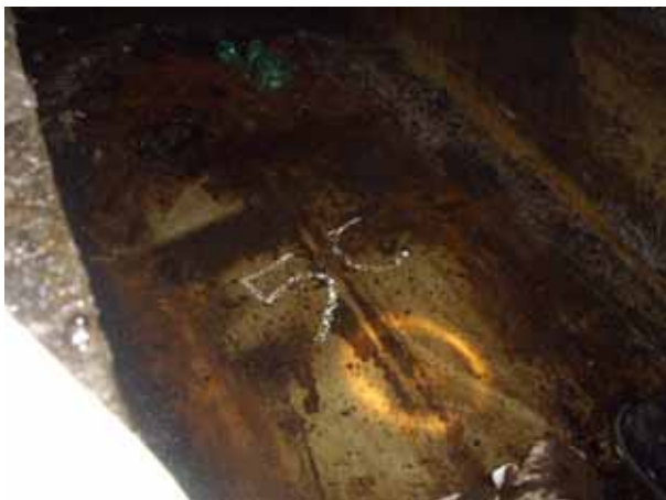
5C Bellmouth underside
