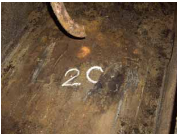
2C Bellmouth underside
