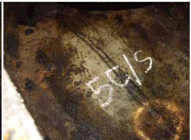
5C stripping bellmouth underside
