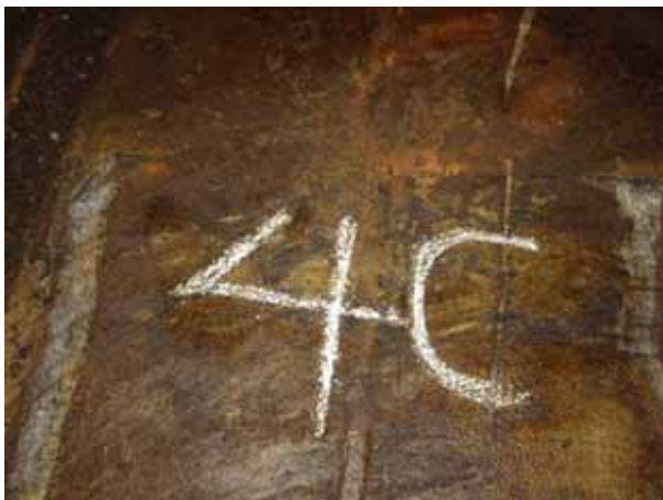
4C Bellmouth underside
