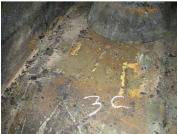
3C Bellmouth underside
