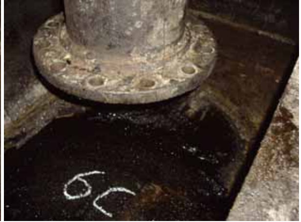
6C stripping bellmouth underside
