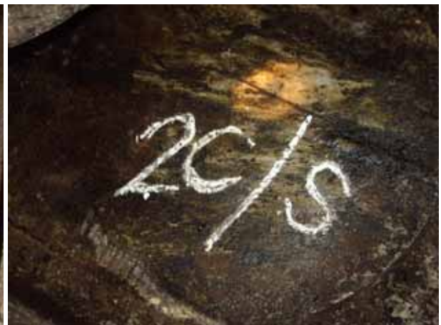
2C stripping bellmouth underside
