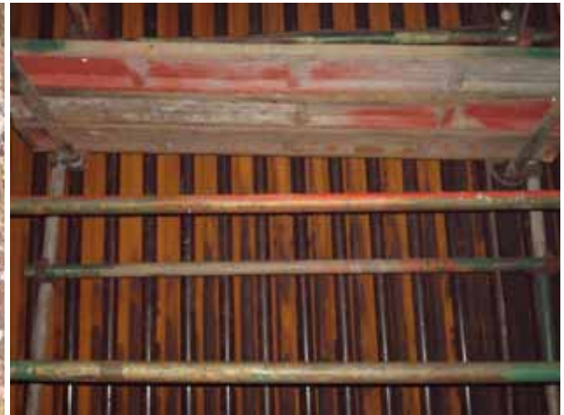
SCREEN TUBE FOR BOILER
