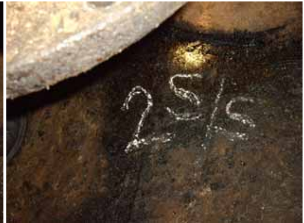
2S stripping bellmouth underside
