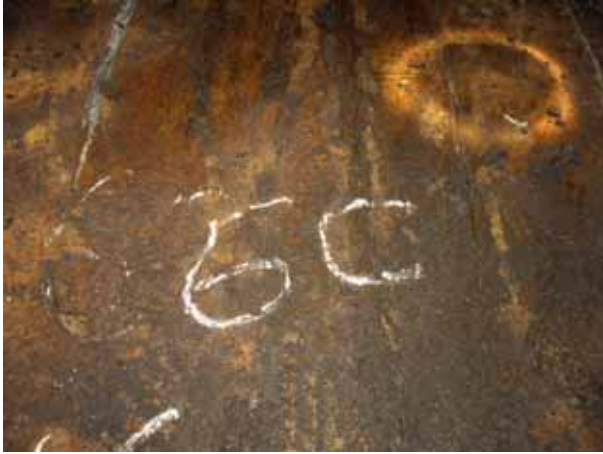
6C Bellmouth underside
