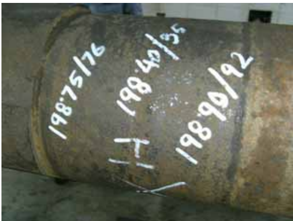
Heavy corrosion on shaft bearing position
