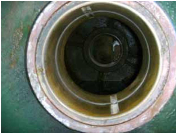
Wire drum bearing housing
