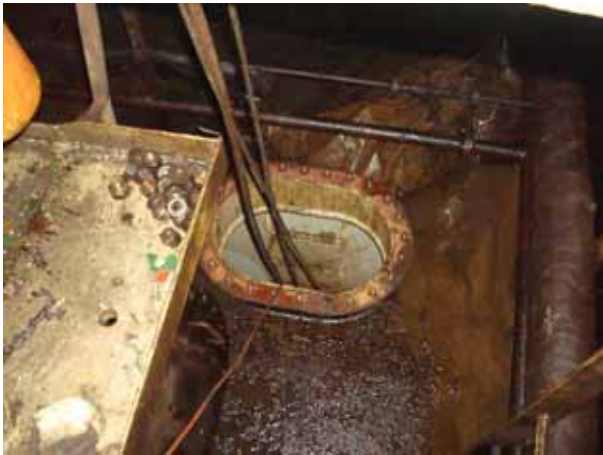
Bilge tank cleaning
