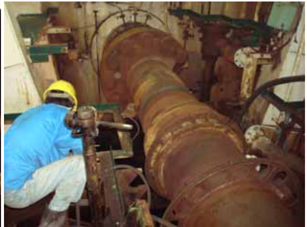
Tailshaft intermediate shaft dismantled
