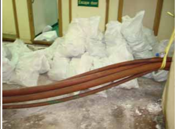
Upper Deck Floor renew
