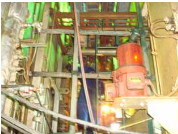
Staging for boiler
