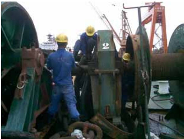
Windlass dismantled shaft with wire drum
