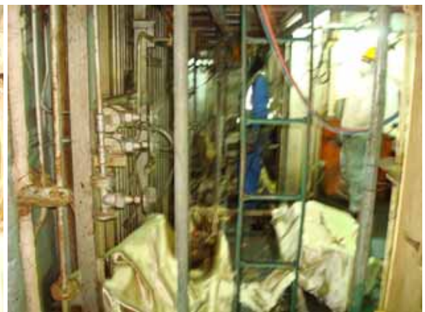
Staging for boiler
