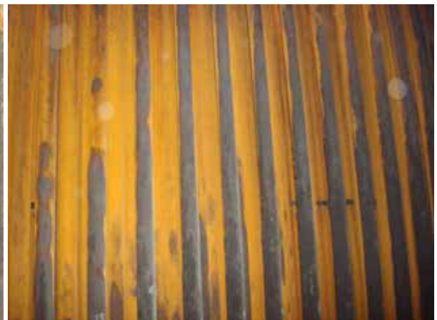
Furnace side Wall tube top side
