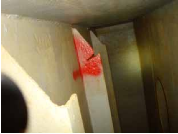
Stiffener crack
