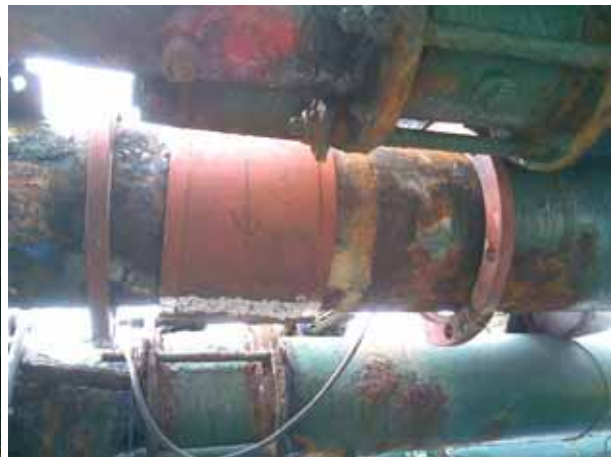
Expansion joint renew for cable pipe
