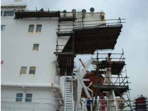
BRIDGE WING STAGING
