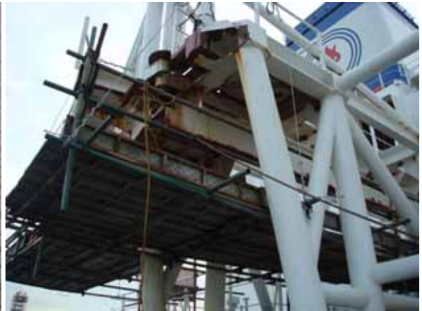
STAGING FOR PROVISION CRANE
