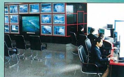
工藝在綫監控系統 Technology online monitoring system
