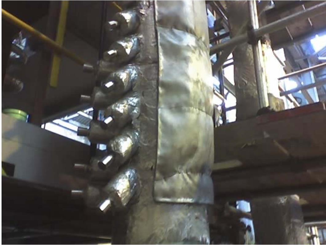
圖2.1.3-5 垂直取樣點(Vertical sampling ports)
