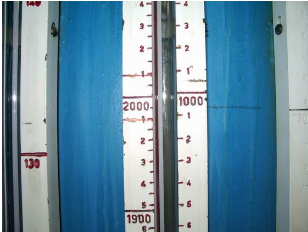
Sight Glass Two readings - tanks are manifolded Badger Meter USA
