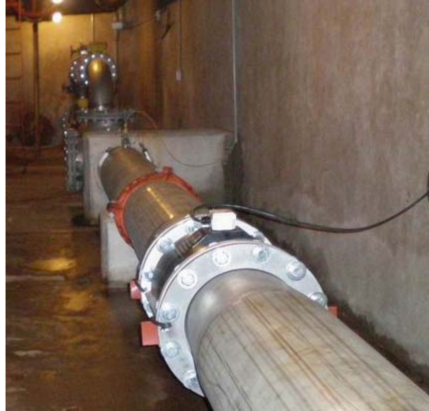
DN 400 Electromagnetic Meter CFB Trenton, Canada
