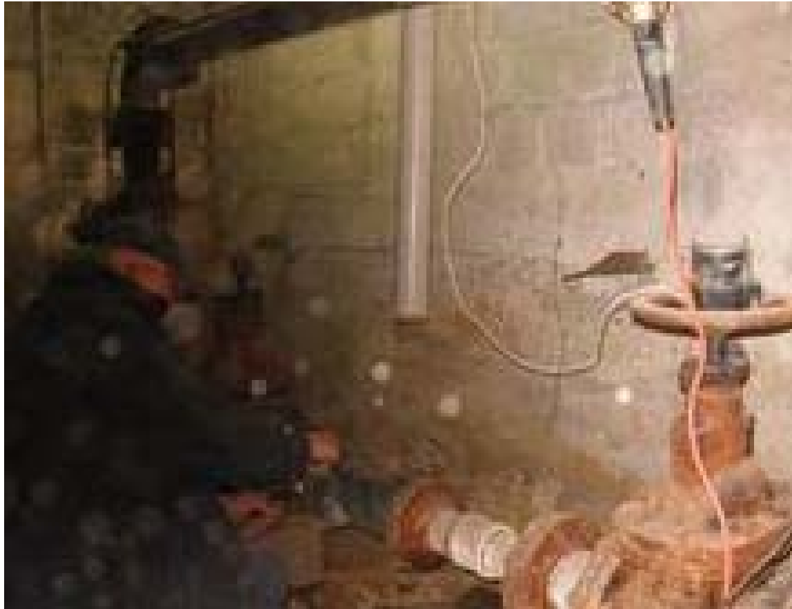
West Quinte, Ontario, Canada Removal of Turbine Meter
