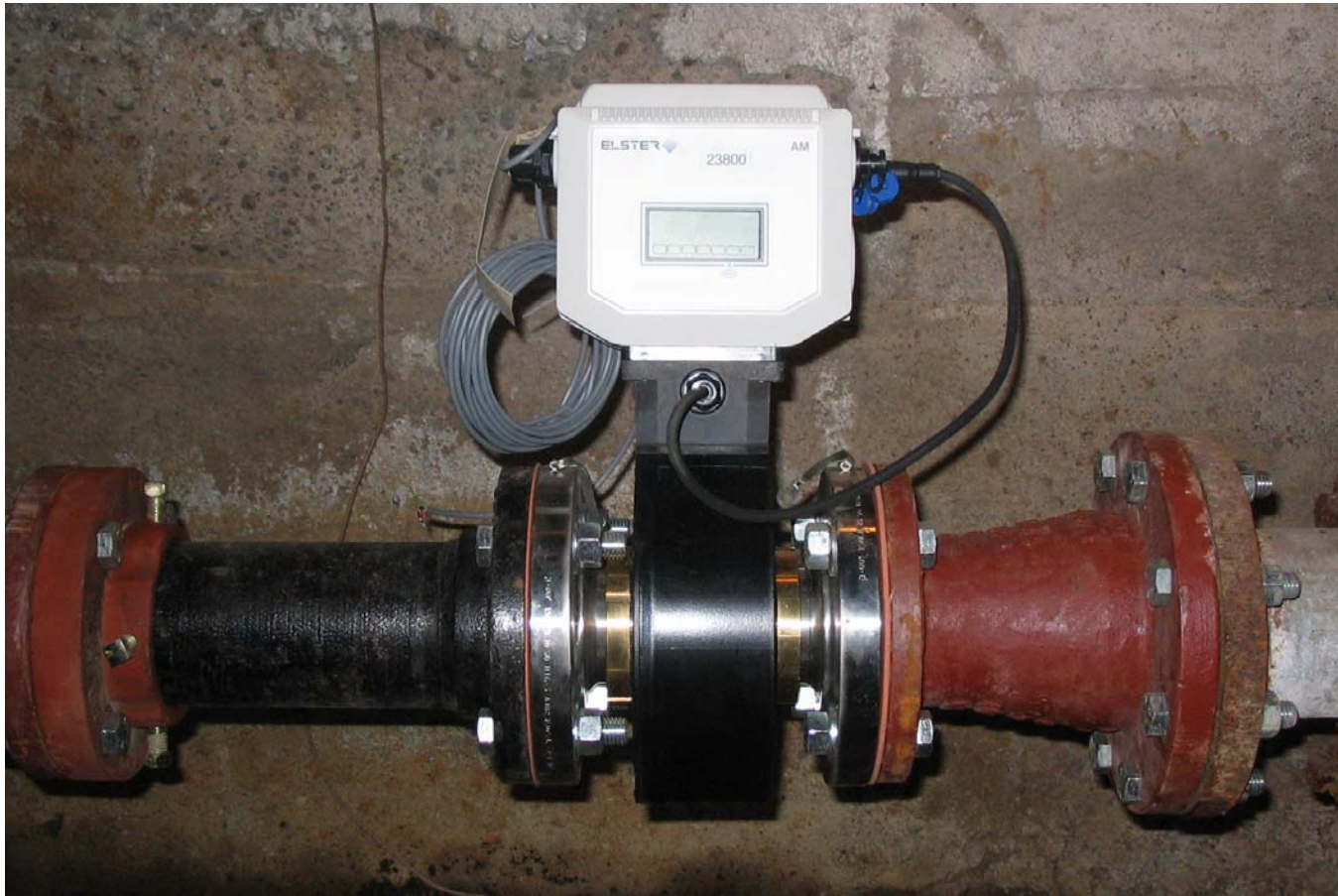
West Quinte, Ontario, Canada Installation of New Electromagnetic Meter
