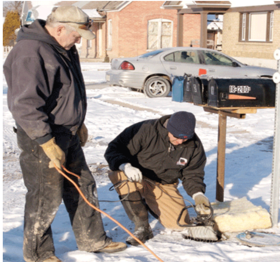
Frozen Meter in Meter Pit Nephi, Utah USA
