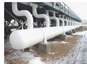
36" dia x 44mm thick gas compression station header inspected using Teletest® to detect corrosion at concrete supports
