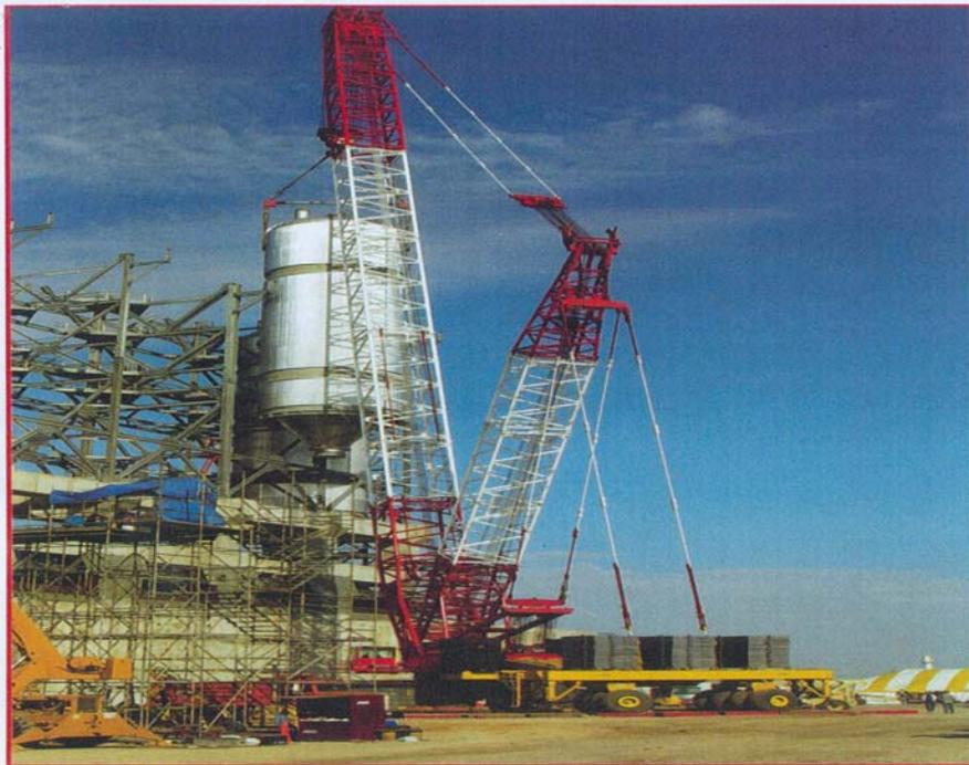
ALE's Liebherr LR1800 crawler crane rigged on superlift using a wheeled dolly to lift into place one of four 320 tonne Coke Drums at Valero site, Texas City, USA.
