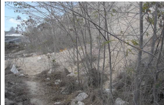
Figure 6 Photo Dust & Overflow from Shore Bin
