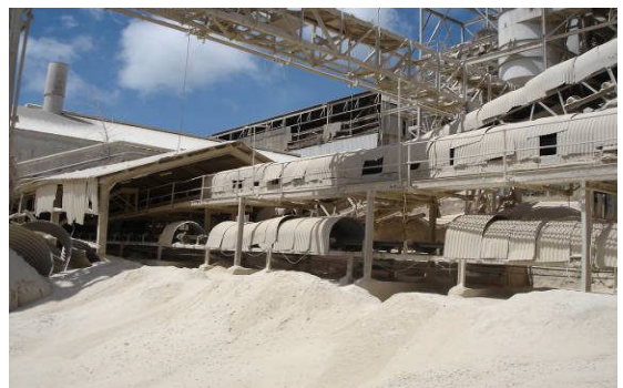
Figure 11 Photo CV D1, & >1.2m deep dust
