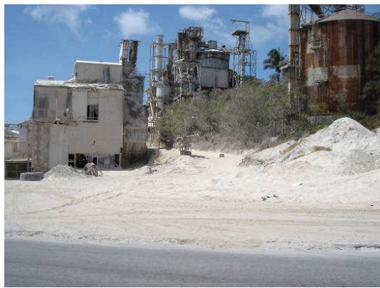
Figure 8 Photo Deposited Dust South of Crusher
