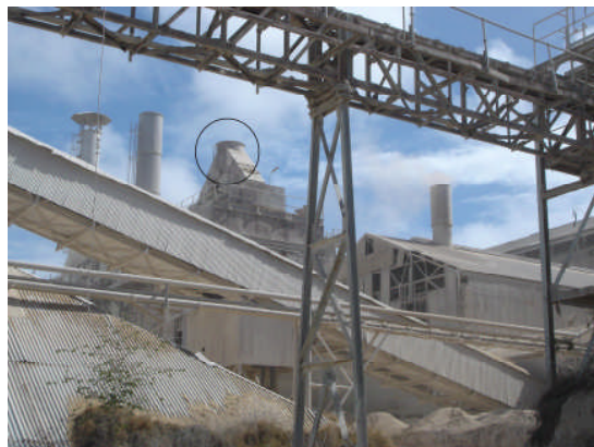
Figure 16 Stack Extension
