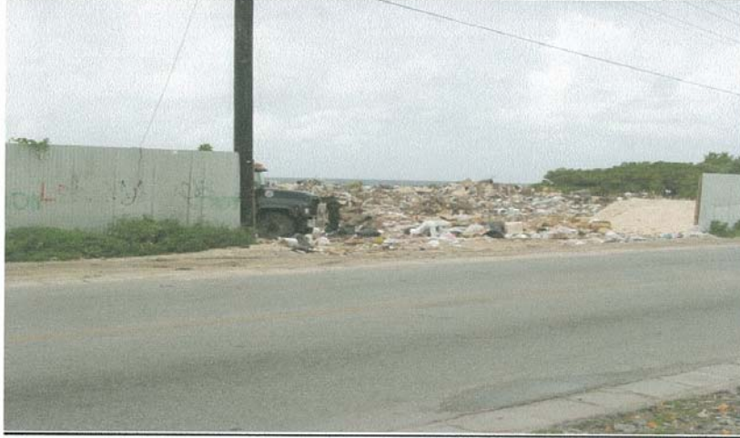
MAJURO LANDFILL ENTRANCE OCTOBER 2006
