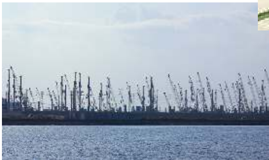
Under construction (Many crane arms)
