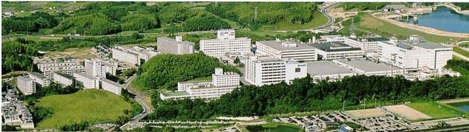
Advanced Development and Planning Center (Tenri, Nara)
