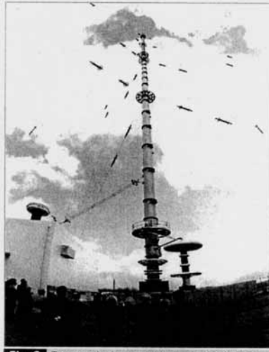
Fig.2 Transmission antenna of 200-m in height (Hagane-yama LF station)
