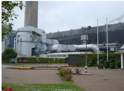
Fiddler's Ferry電廠新設置的排煙脫硫設備及生質燃料輸送帶
