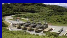
Biogas power plant, Municipal waste landfill, Taipei
