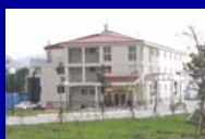
RDF demon plant in Hualien BOE Project, Tech. developed by ITRI
