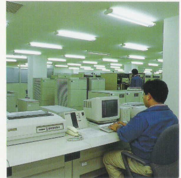
RDP Computer room
