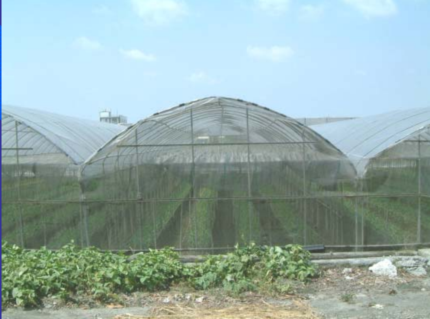
D. Simple galvanizing steel greenhouse
