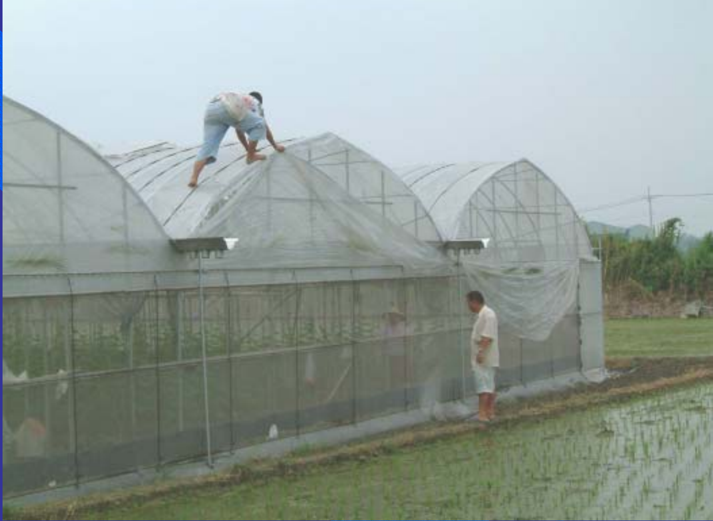
C. Simple galvanized steel with T type reinforce structure Greenhouse :
