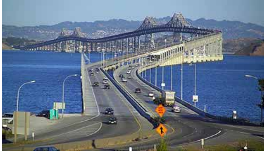
Richmond-San Rafael Bridge
