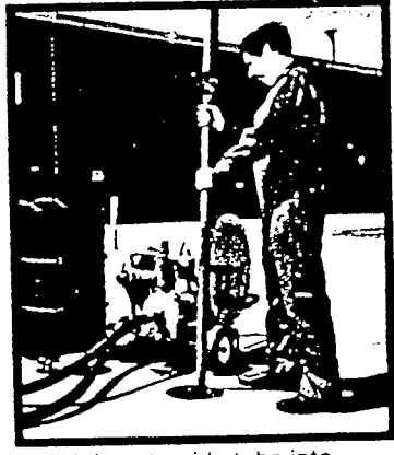
4. Insert guide tube into storage tank.
