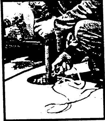
7. Attach ground wire clip to tank.
