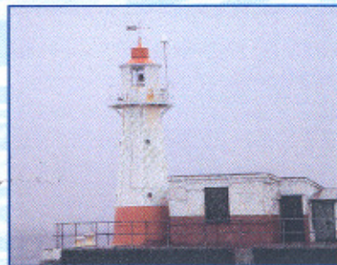
The Newlyn tide gauge site. Newlyn was used to determine UK mean sea level. It is the benchmark for the whole of the United Kingdom, that is, all heights are referenced to this point.
