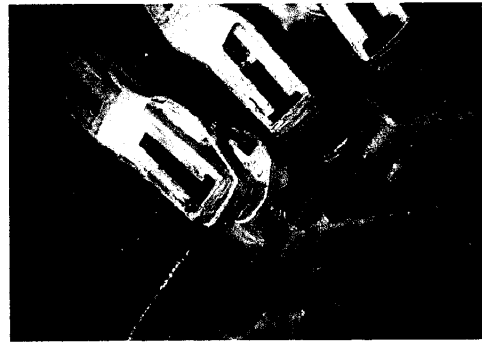
FIGURE 4 - Final installation of the sensor head and optical cable with same integrated material used to brace the end-windings
