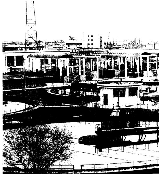
An imposing picture: The turnkey sewage plant at Hangzhou, People's Chinese Republic, built by PASSAVANT-ROEDIGER.
