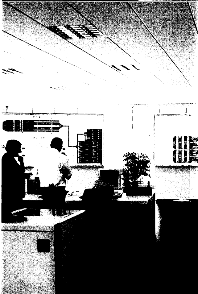
Process visualisation with large screens at the central control room of the Wiesbaden main sewage works.
