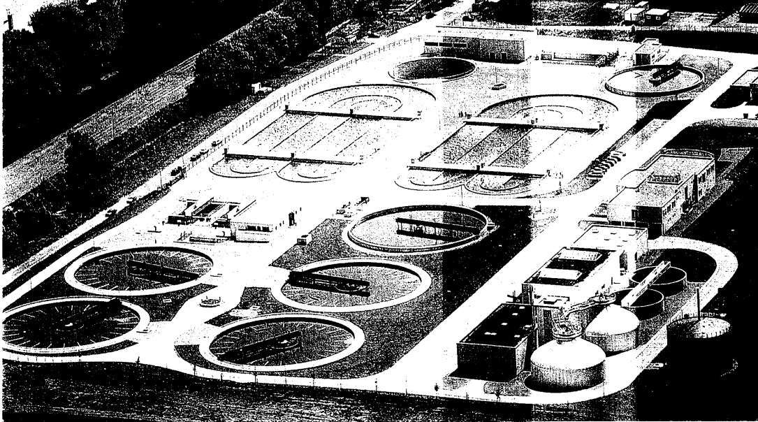
The Gotha central sewage plant (picture above) for 150,000 P.E. set up by PASSAVANT-ROEDIGER as turnkey complete solution in only 24 months.
