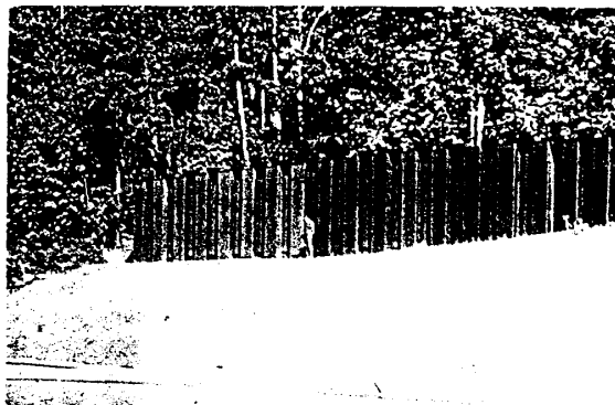
Wooden Noise Barrier
