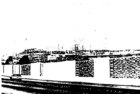
Masonry Noise Barrier
