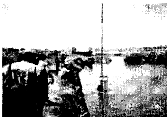
Fig.9 Dismantling Illegal Wells in I-Lan County
