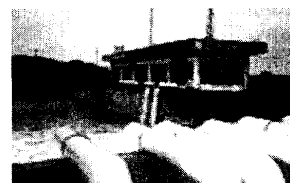
Fig.7 Ta-Wen Salt Water Supply Factory in I-Lan County
