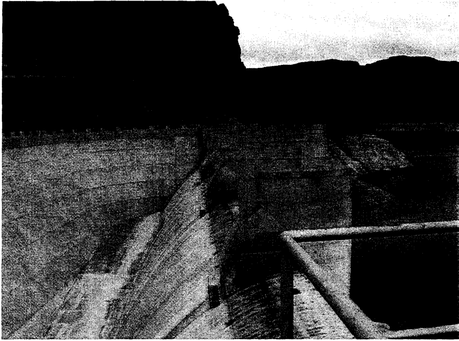
Hoover Dam 右岸溢流堰
