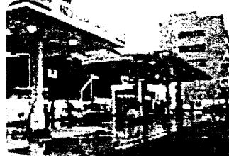
Natural gas Eco-Station
