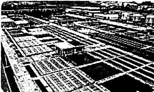
Photovoltaic Power Generation at the Murano Water Purification Plant, Osaka
