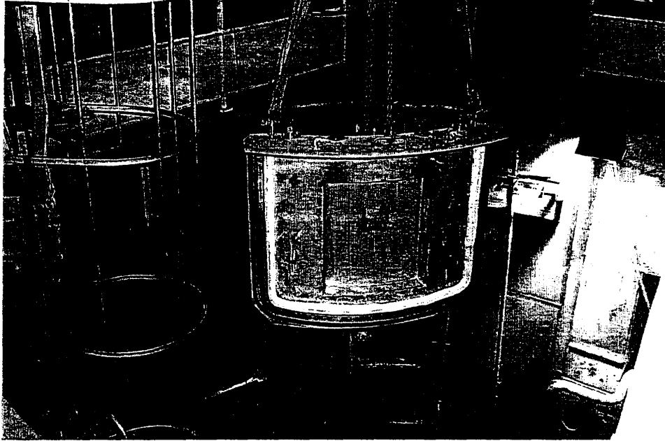
Picture 1: Actual installation of the sealing device.
