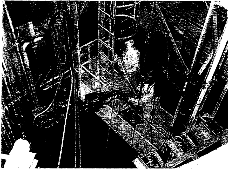
Figure 36: Cutting tool during maintenance (lower level of the mobile footbridge)
