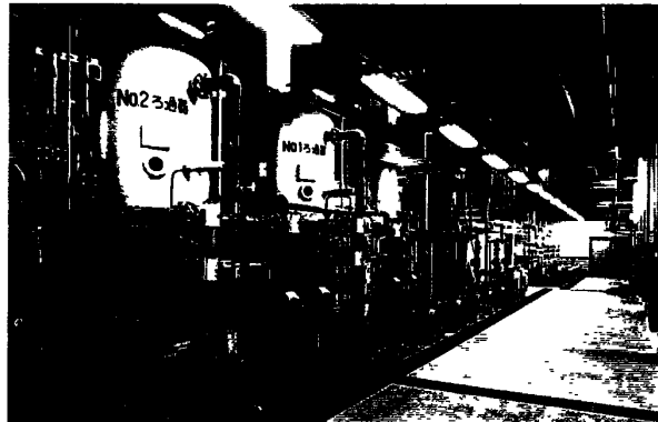
排水処理設備 Waste water treatment system
