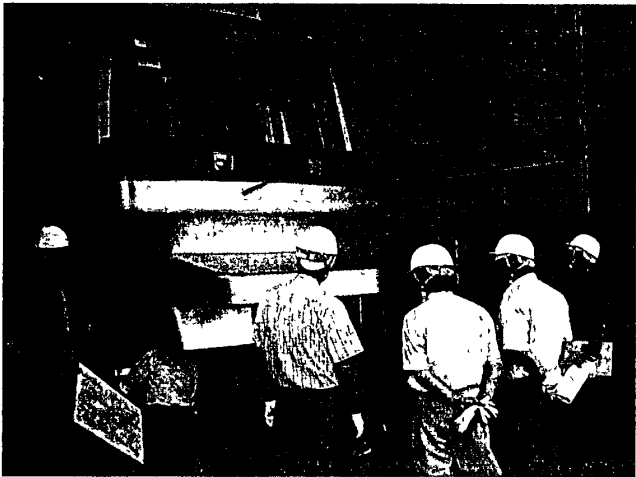
DIMENSION MEASUREMENT OVERALL LENGTH OF No 12 CAR
