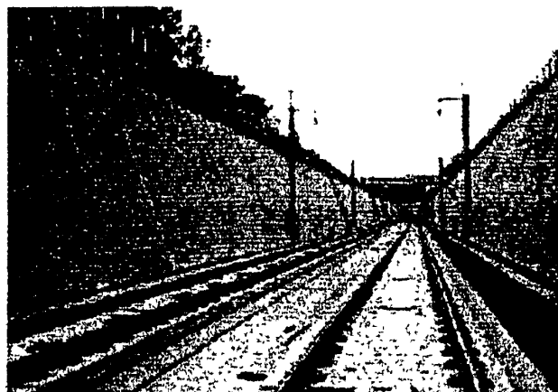
Figure 8 RCRS laid on cutting along the Hokuriku Shinkansen line
