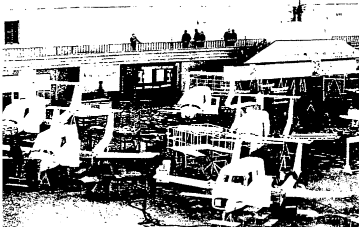
Assembly shop of AVIAKOR airplane plant in Samara
