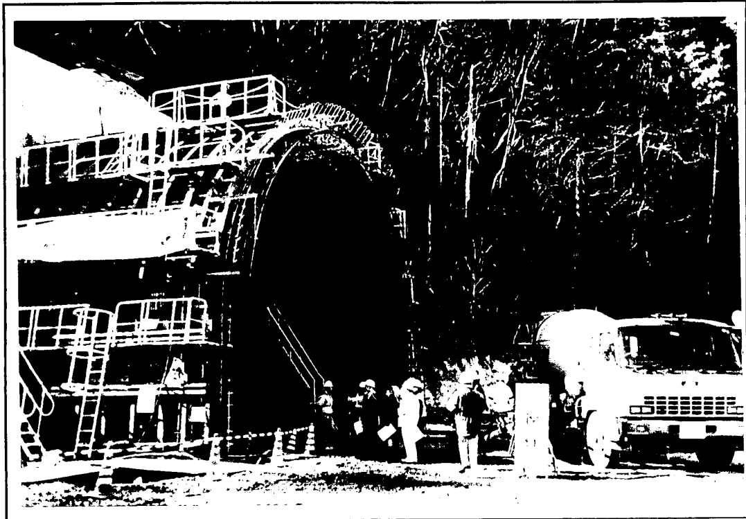
洞口處之施工
