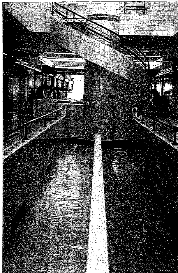
The filtration room
