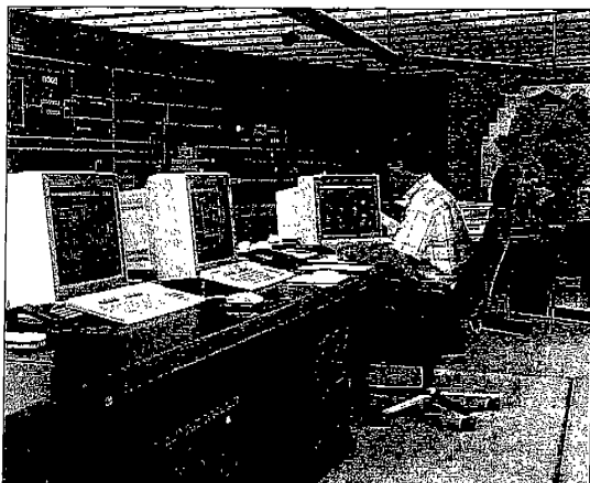
The central control room
