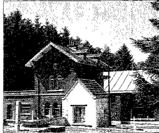
Braine-l'Alleud. Pumping plant of La Vau
