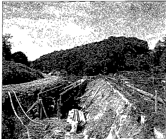
Crupet. Altering the brook of Assesse into a strait to protect it against floods.
