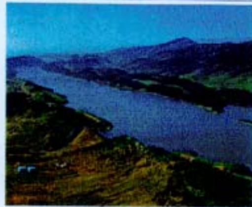
Horseshoe Dam and Reservoir
