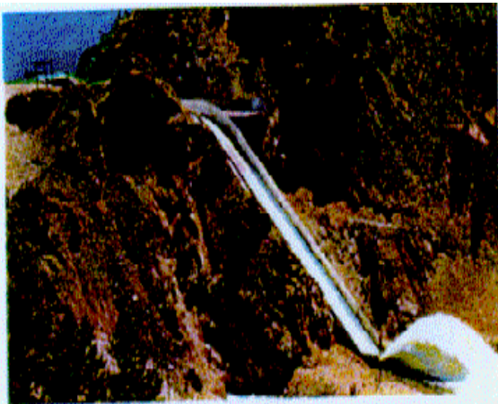
Spillway at Granby Dam
