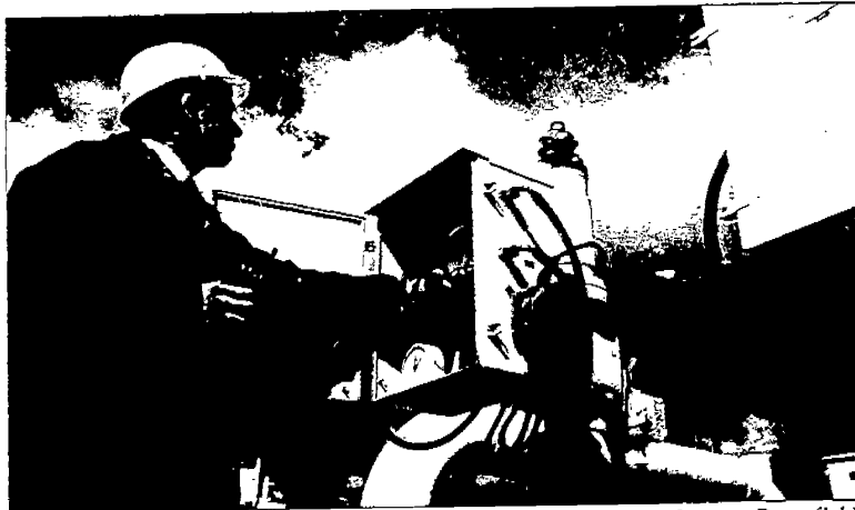
A BPA engineer adjusts the control unit for an hydraulic valve at Buncefield, northwest of London. The valve is operated and controlled via the new scada system from Kingsbury near Birmingham, 100 miles north. (Photograph by John D. Elton.)
